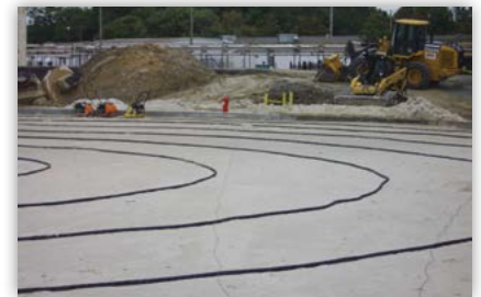
MATCOR Tank Ring SPL-Anode installation
